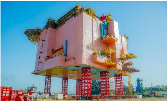
Figure 4: BorWin6 offshore converter platform (topside) at Jebel Ali Port in the UAE. Credit: McDermott [5]
